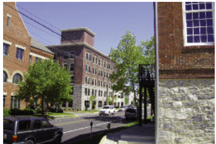
Winchester block with new office building, restored Knitting Mill, and new parking garage.
