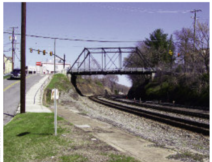
Saved by innovation: Knowing the historic Hawthorne Street bridge was important to Covington, VDOT and Virginia Tech developed a lightweight deck that could keep it in service.
