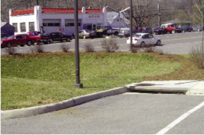
This Lexington Firehouse parking lot drains to a specialized media that removes oils and other pollutants.
