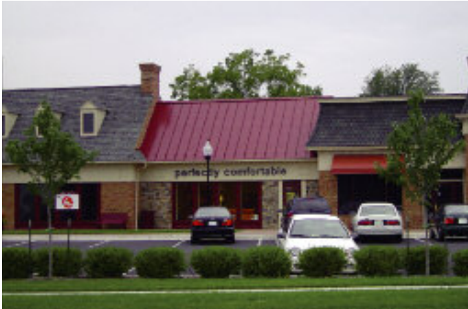
Landscaping along the road screens this Winchester parking lot from view.
