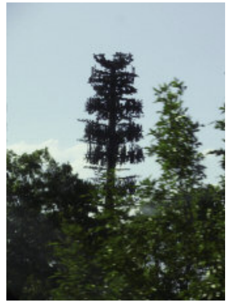
Communications tower disguised as a tree, New Jersey
