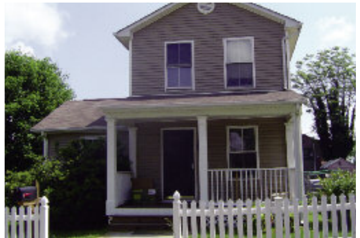
Habitat for Humanity project, Lynchburg
