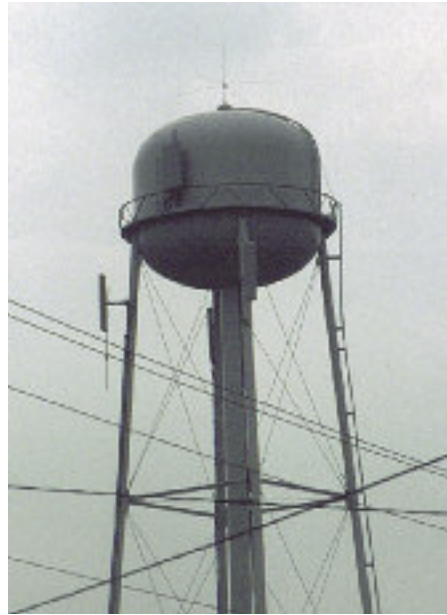
Co-location on water tower, Rockingham County
