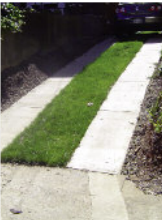
Driveway strip uses less pavement (Staunton).
