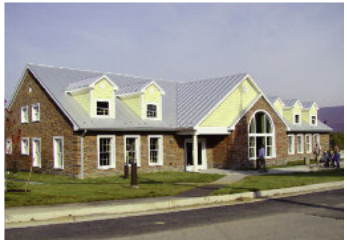
Library in downtown New Market, designed for energy efficiency and featuring reused materials, permeable pavement, and rain gardens
