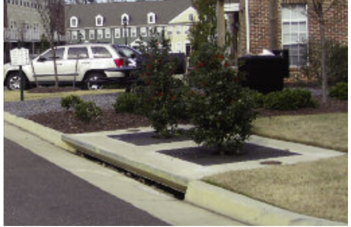
Multiple smaller facilities like this tree box filter reduce runoff and filter pollutants (Williamsburg).
