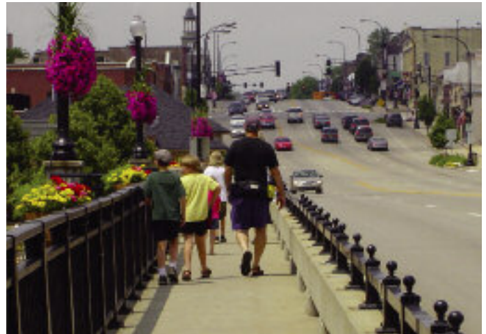
Safe, convenient sidewalk on the bridge enables pedestrians and bikers to cross the Fox River in Geneva, Illinois.
