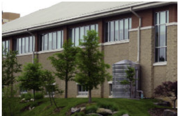
Large-scale rain barrel collects runoff for reuse (Arlington).
