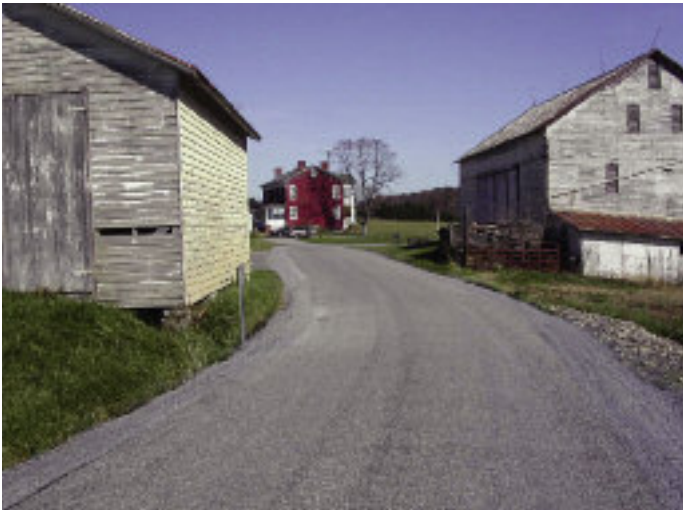
The Rural Rustic Roads program allowed this road in Augusta County to receive repairs without widening.
