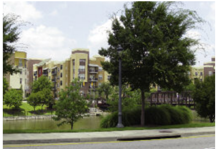
Atlantic Station, Atlanta, where residents and workers drive less
