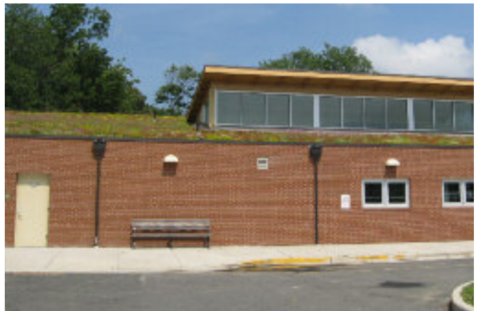
Green roof absorbs rain at an Arlington community center.
