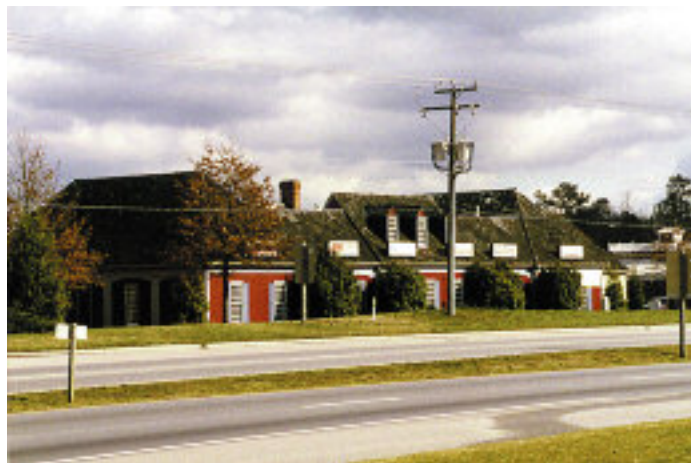
Parking hidden, Chesterfield County
