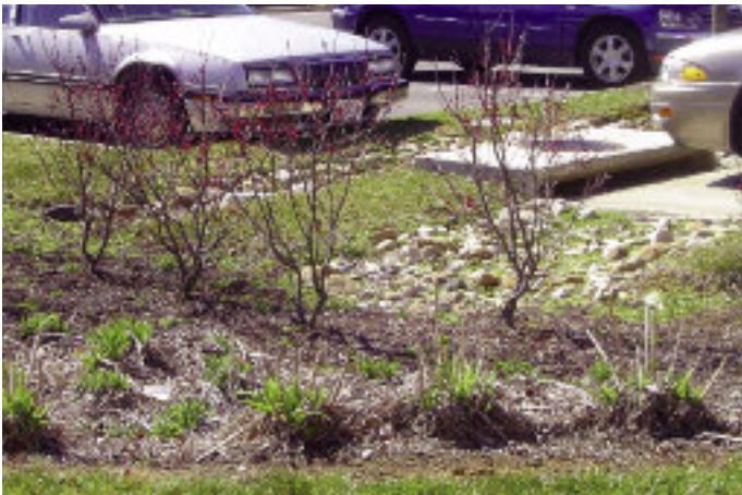
Parking lot drains to a rain garden at Kendall in Lexington.
