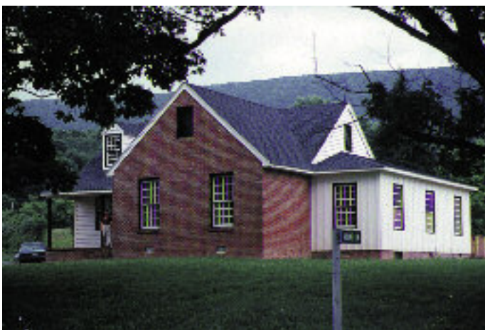
Office made from pre-manufactured units, Bath County
