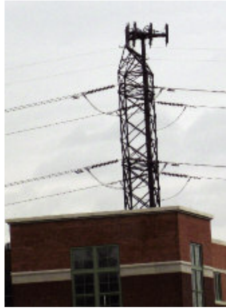
Co-location on office building, Albemarle County
