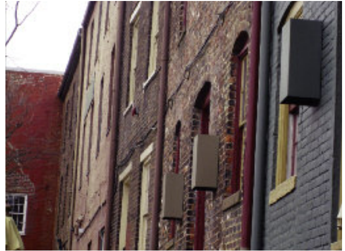
Shielded lights on historic buildings in Staunton
