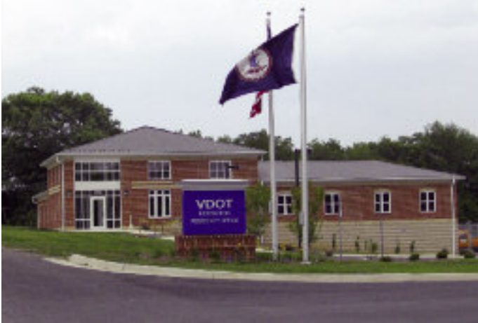
VDOT Residency, Rockbridge
