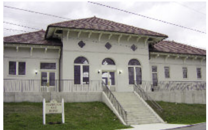
Individually listed on the National Register: Covington Depot
