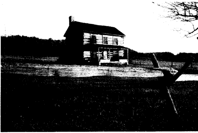
Log house, Silverbrook Farm, southeast of Middlebrook. Dating to the 1850–1890 era, the house is an example of the mid-19th century hall-and-parlor plan, a popular architectural form in the Corridor.
