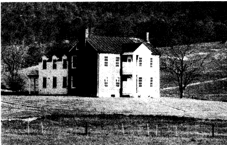
G.W. Brandenburg House, Summerdean area. Built ca. 1834–1836, this brick I-House is adorned with a two-tiered entry porch, a classical feature.
