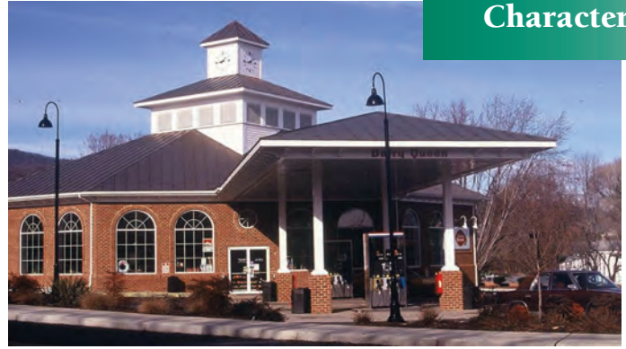
Amoco canopy and building in traditional materials, Crozet
