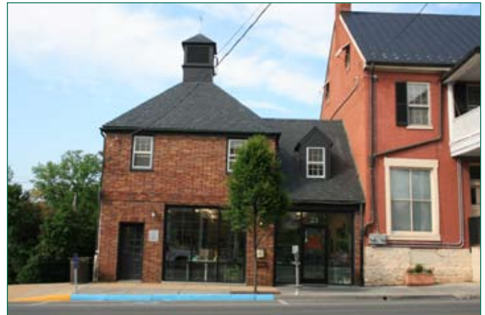
Fire House Gallery and Shop, Town of Berryville
